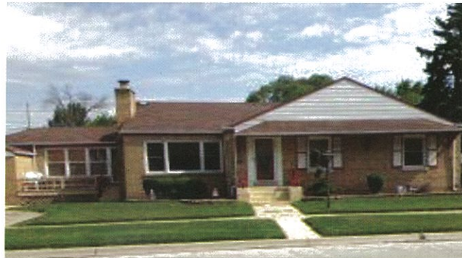
Meets the property maintenance codes
